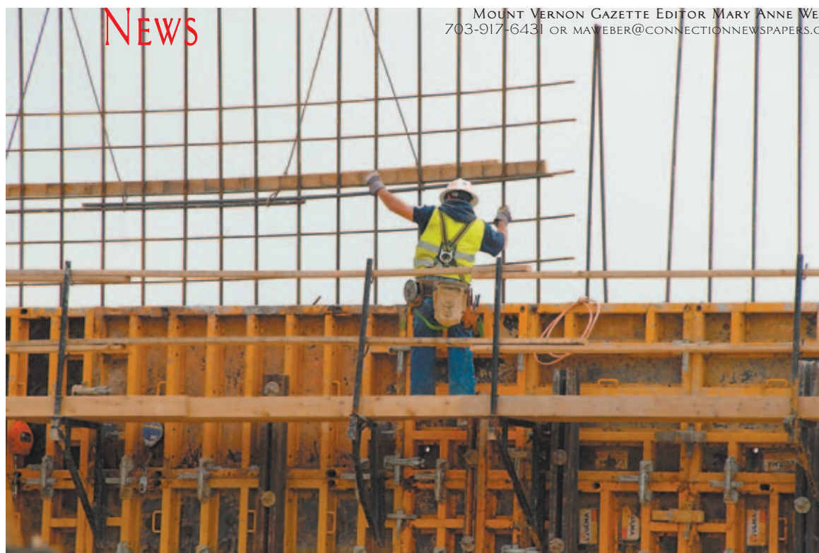
A rodman installs reinforcing steel on the technical building exterior wall.
