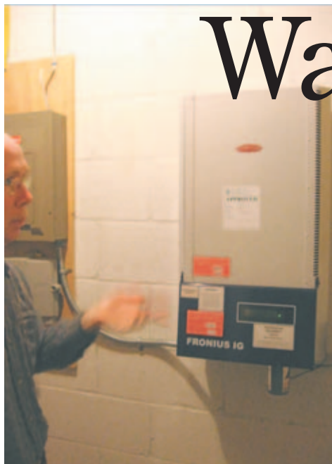
Richard Watts points out the converter box where his solar electricity is changed from direct to alternating current.
