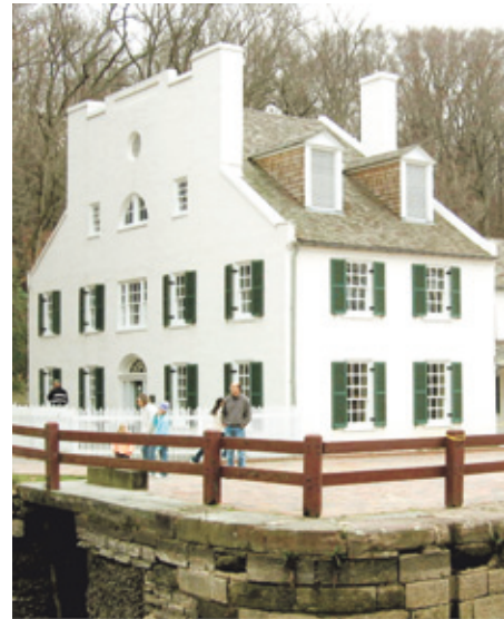
Great Falls Tavern reopened earlier this year after renovations to the historical building and its visitor center.
