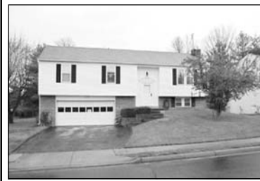
Burke $414,900 Welcome home to Cardinal Glen. This home has it all: size, 3 bedrooms on the upper level, office/guest room on the lower level, private swimming pool, location, and schools. The rec room is highlighted by a wood stove and updated windows. Richard Esposito 703-503-4035
