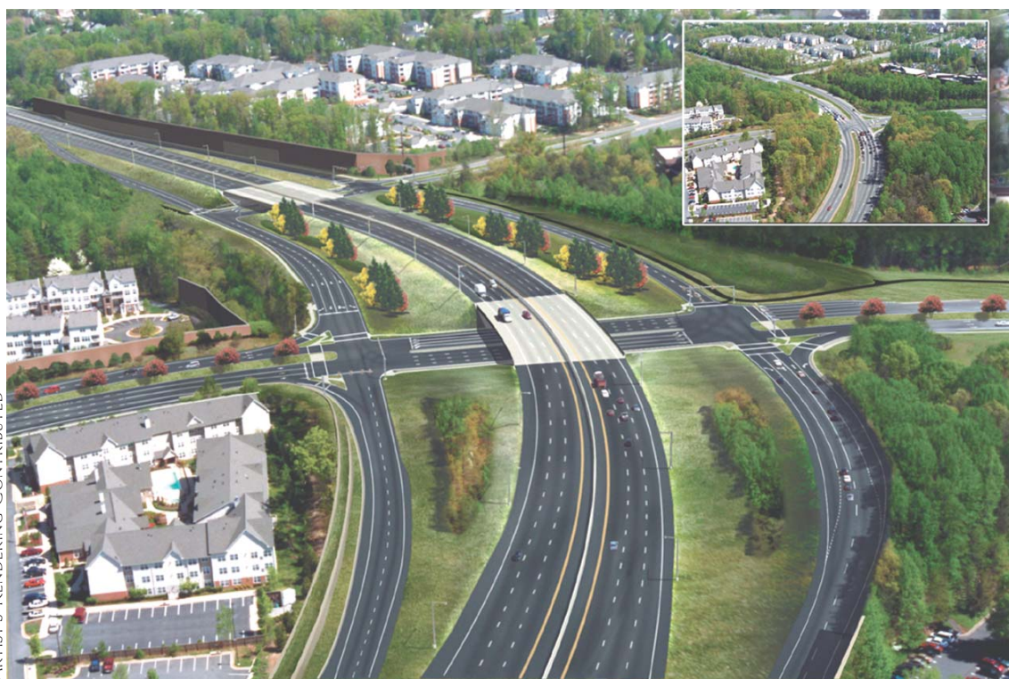
Construction should begin on the interchange at Fair Lakes and Fairfax County parkways in 2010 and take about 2 1/2 years to complete. For project details, see www.connectionnewspapers.com , click on Centre View.
