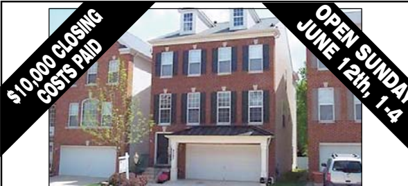
Mt. Vernon/ Ft. Belvoir $525,000
