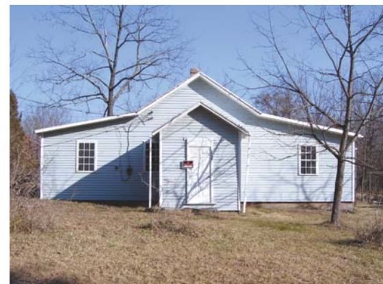
West facade looking east. PHOTO BY PAT LAYDEN
