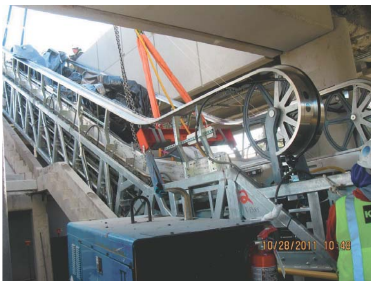
Escalators being installed at Wiehle Avenue station.
