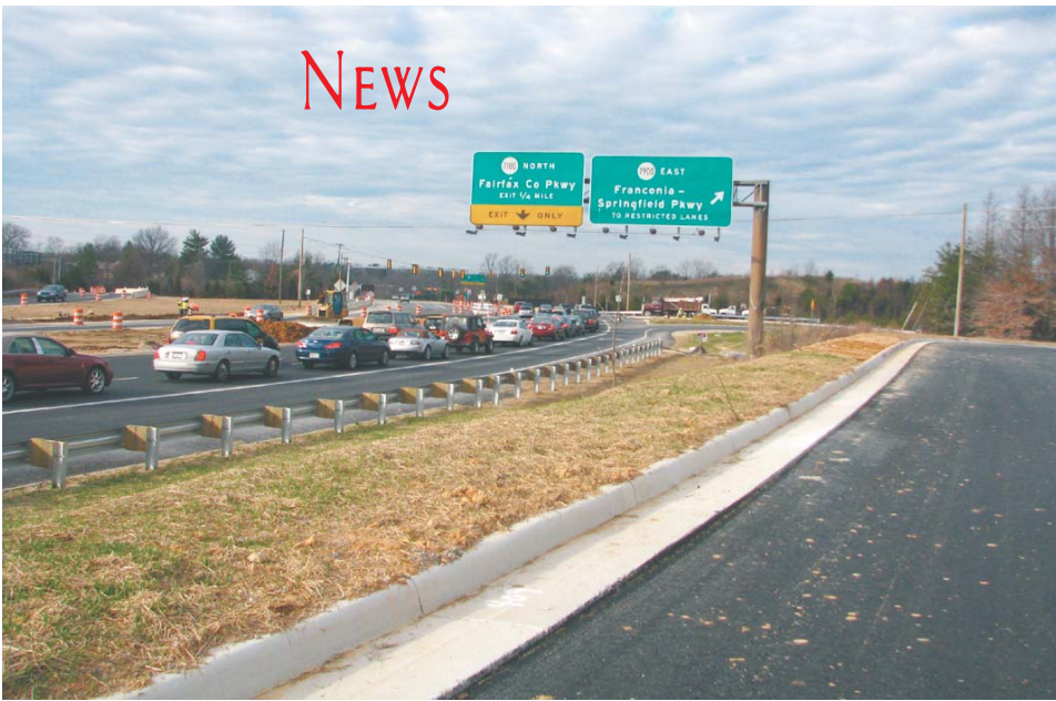
PHOTO BY MIKE SALMON/VIRGINIA MEGAPROJECTS
