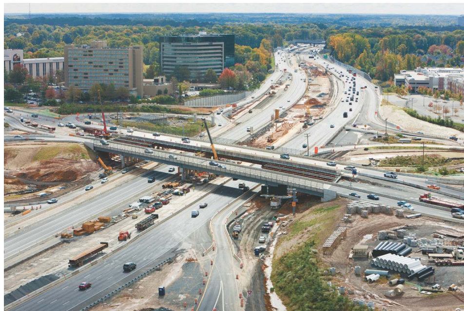
The new Route 7 overpasses take shape over the Capital Beltway.
