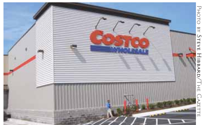
The new Costco will open to the public Thursday, Aug. 8, along Route 1 next to Wal-Mart.
