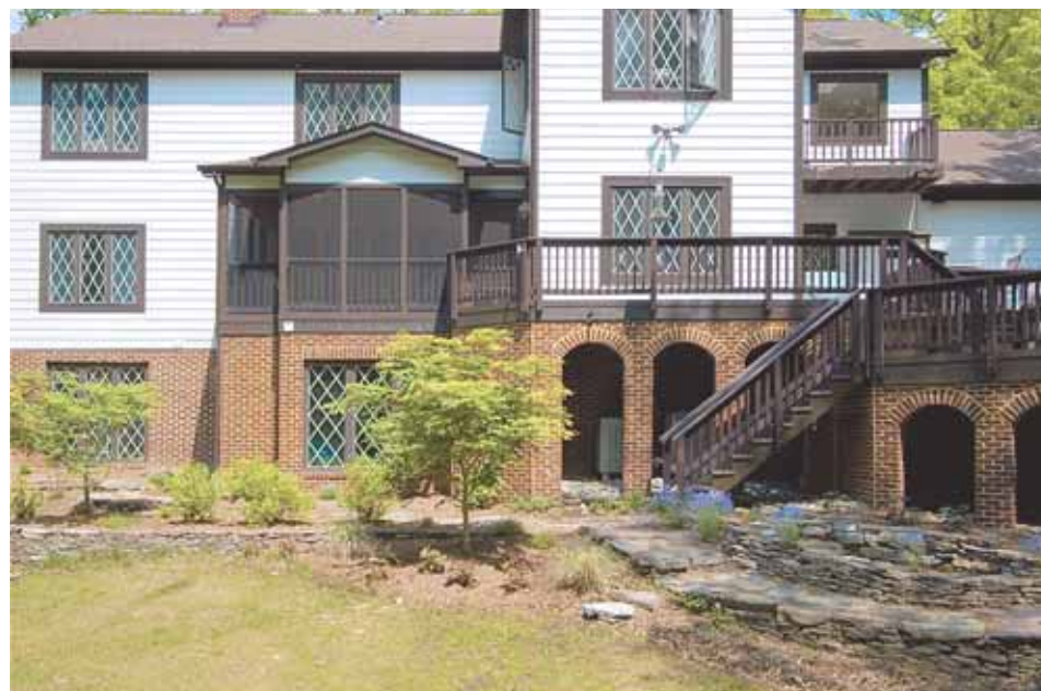
PHOTO COURTESY OF FOSTER REMODELING SOLUTIONS
