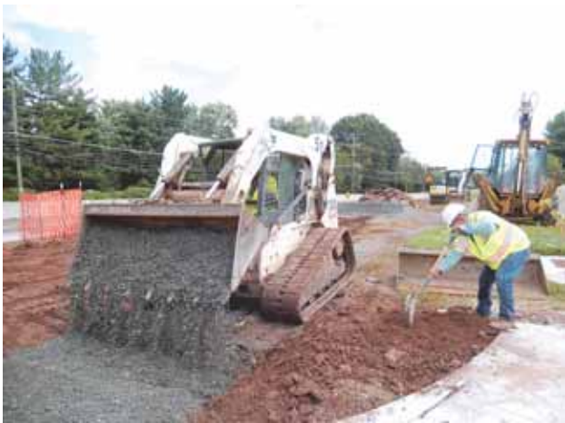
Workmen across from Rocky Run Middle School create what will be an asphalt bicycle-and-pedestrian trail along Stringfellow Road.
