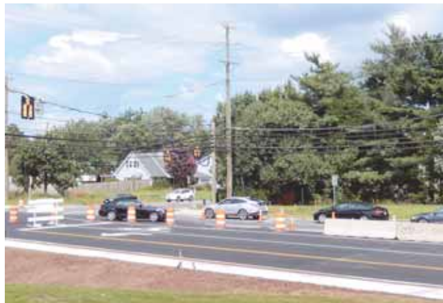
Southbound motorists are directed onto the old section of Stringfellow Road, while northbound traffic drives beside the new portion not yet open.
