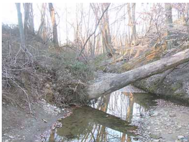
Stream erosion in Quander Brook undermining trees along the banks.
