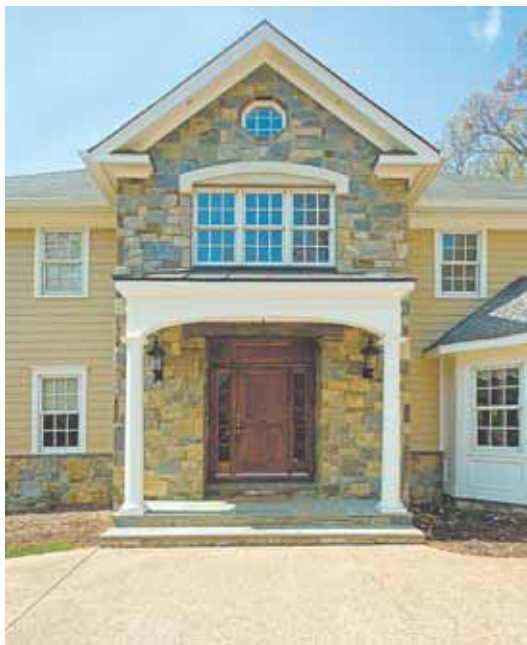
The new portico lends needed definition to the entrance way of the Jeff and Sharon Roman’s Great Falls home. The metal-clad roof is visually unified with a garage overhang supported by decorative brackets.
