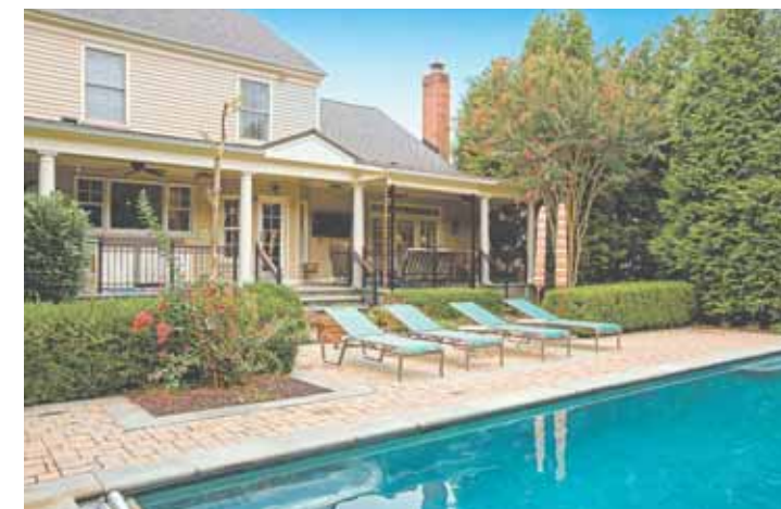
To create the shady spot appropriate for dining, Jeremy Fleming extended the shed roof which is now covered with an architecturally-appropriate seamless metal.
