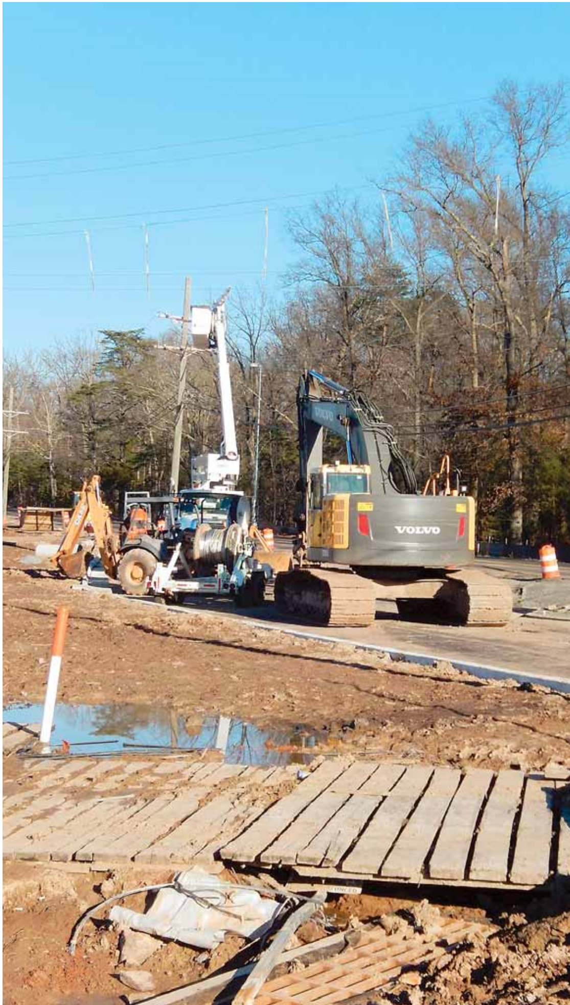
Construction equipment stands at the ready along Pleasant Valley Road.
