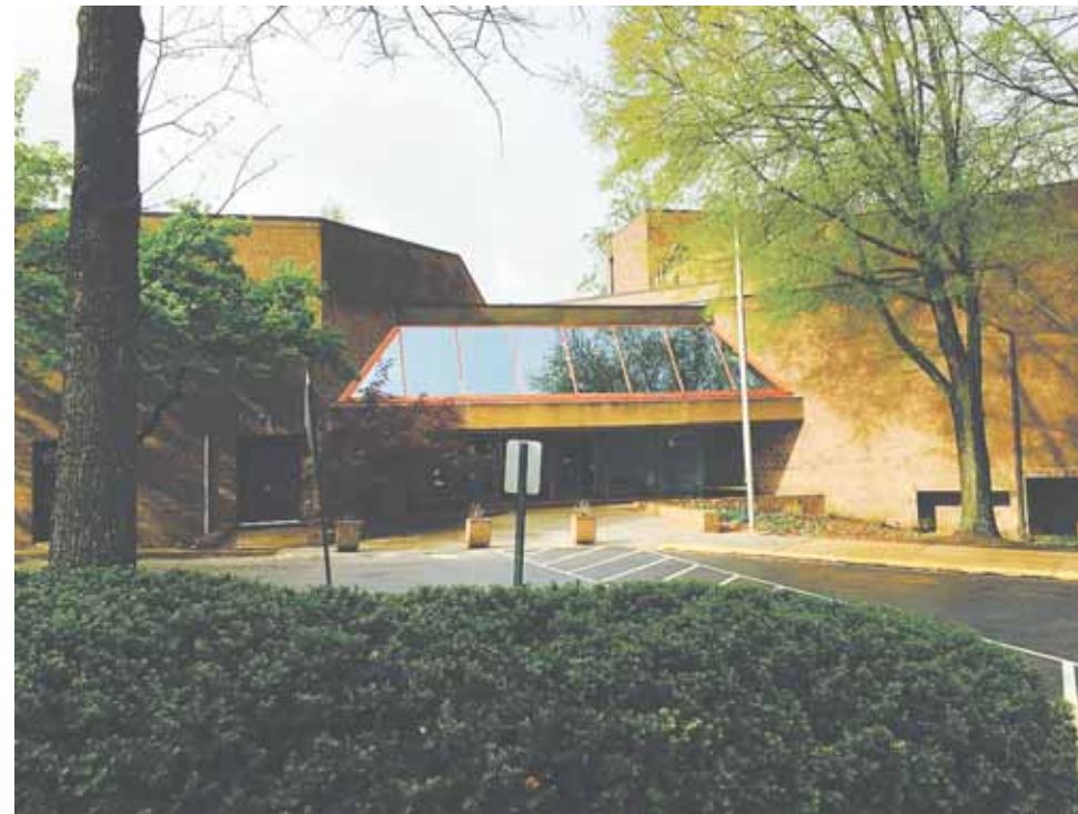
Construction on the McLean Community Center's renovation is anticipated to begin in the fall of 2016.
