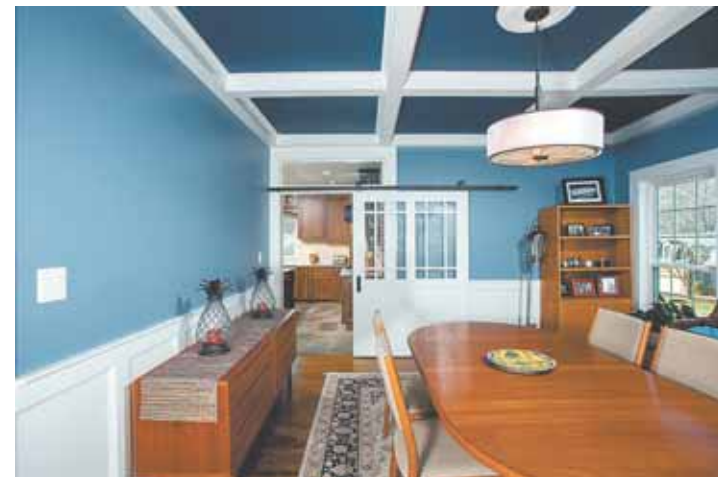
With its coffered ceiling and Wedgwood interior treatment, the dining room explores 18 th century (Colonial-era) themes. The circa-1890's glass-and-wood barn door mounted on rollers was created by Sun Design. The innovation provides privacy, yet allows light from the home's west-facing rear elevation.
