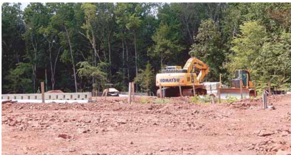
Preliminary site work is underway at The Preserve at Westfields.
