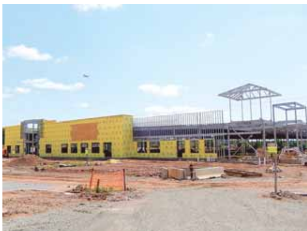
The Wegmans store in Chantilly is under construction on Newbrook Drive.
