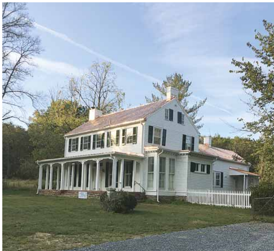
The Darby House behind Seneca Store is also planned for rehabilitation and future lease. The roofing has already been replaced.
