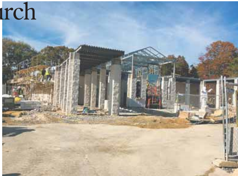
Lots of work underway at St. Lawrence Catholic Church.
