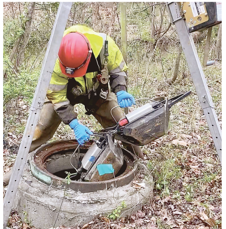
Matthew Moss lowers equipment into system
