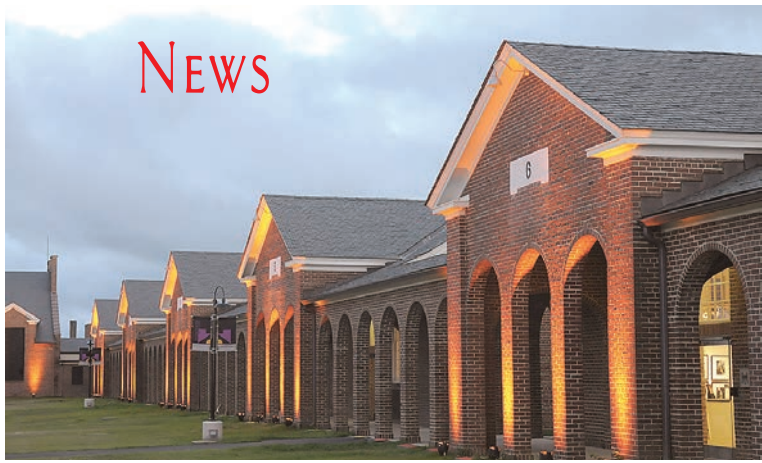
PHOTO COURTESY WORKHOUSE ARTS CENTER
