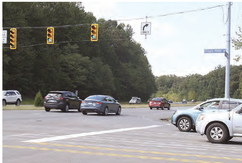
The intersection of the Fairfax County Parkway and Popes Head Road is a focal point of one of the four projects.
