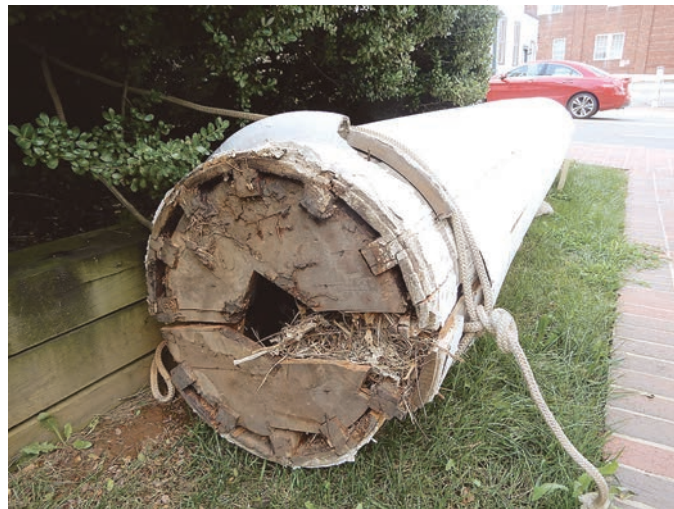
A look inside the top of the pillar, where birds had made a nest.
