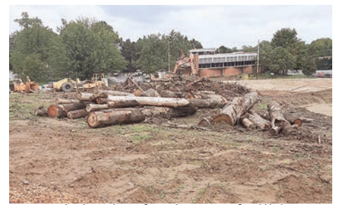
Ground clearing for the new facilities began in July.
