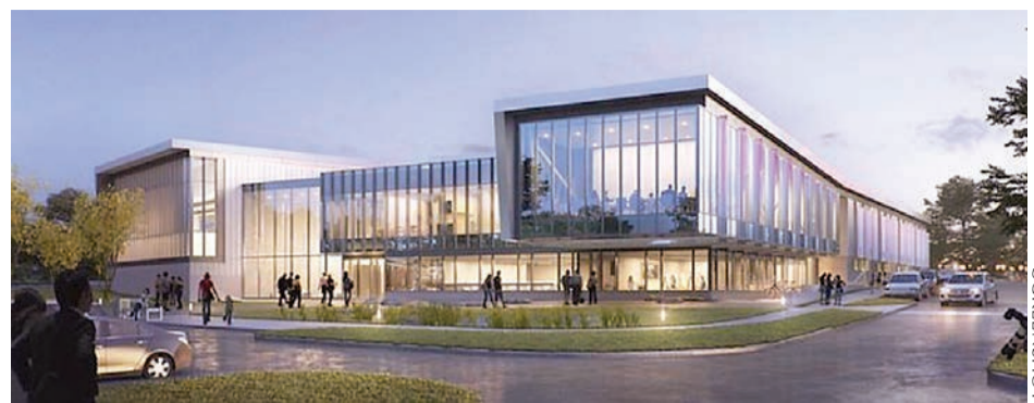
Artist rendering of the proposed building design for The Floris Conservatory of Fine Arts & Music.
