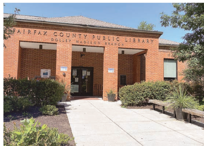
Dolley Madison Library at 1244 Oak Ridge Avenue, McLean is a renovated light-filled building designed and constructed under the U.S. Green Building Council's Leadership in Energy and Environmental Design program. As of Sept. 26, 2020, the library offers virtual children events and adult book talks.
