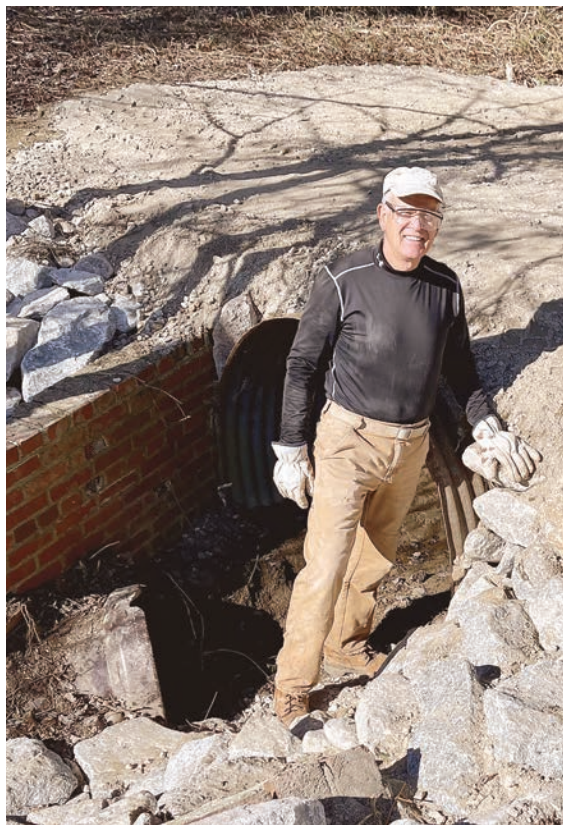
Laurel Hill Park volunteer Michael Applegate stands at his hand dug rock wall lining creek drainage.
