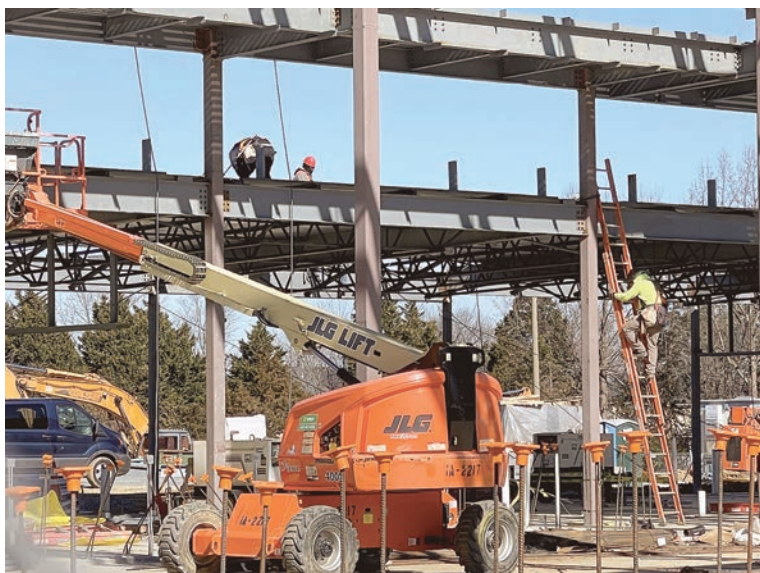
Construction workers place beams using crane and lifts
