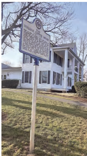
The Coffey house is now being used by Burke Centre for community activities.
