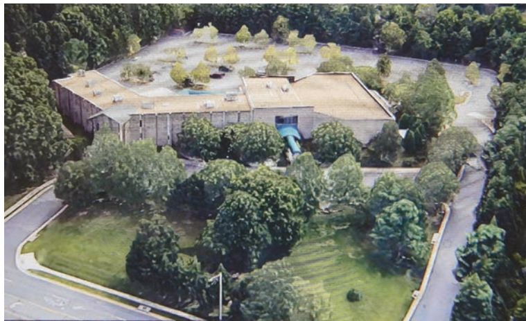
Aerial view of the Fairfax Church of Christ.
