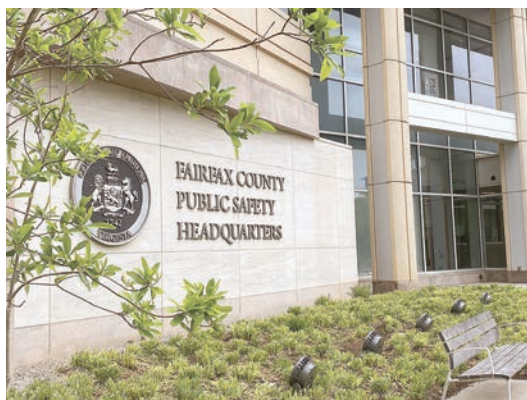
PHOTO BY MERCIA HOBSON/THE CONNECTION Fairfax County Public Safety Headquarters
