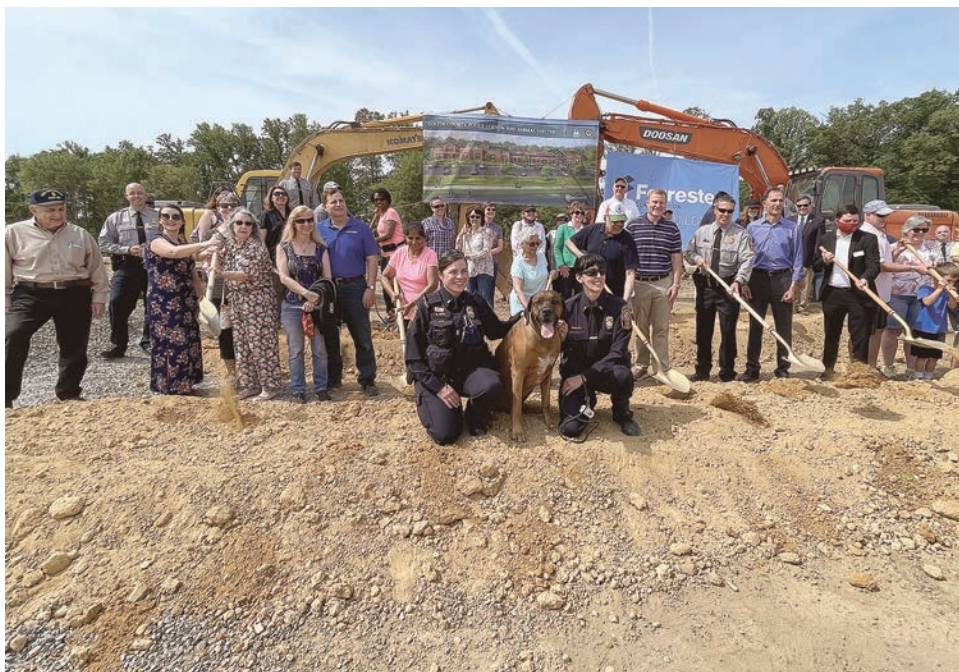
Community members join police and county officials in the official ground-breaking in Lorton.
