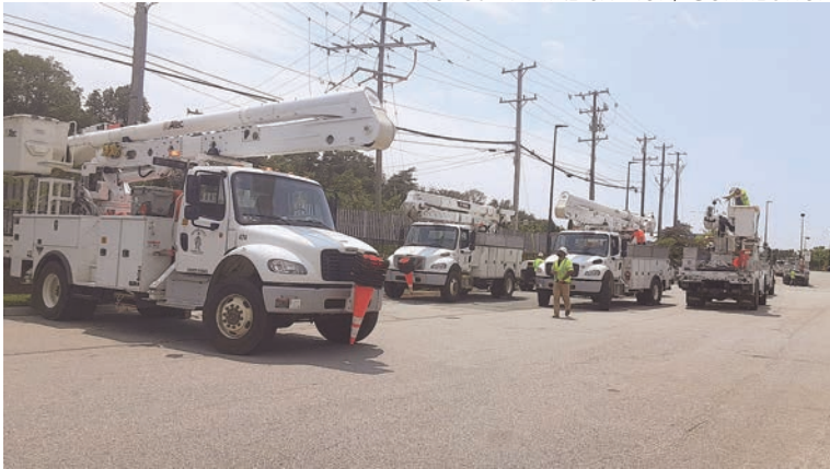
Undergrounding the wires has a lot of advantages.
