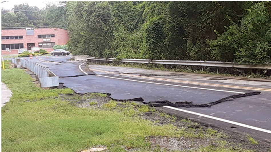
Water overflowed the banks of Long Branch and damaged newly-paved Newington Road.
