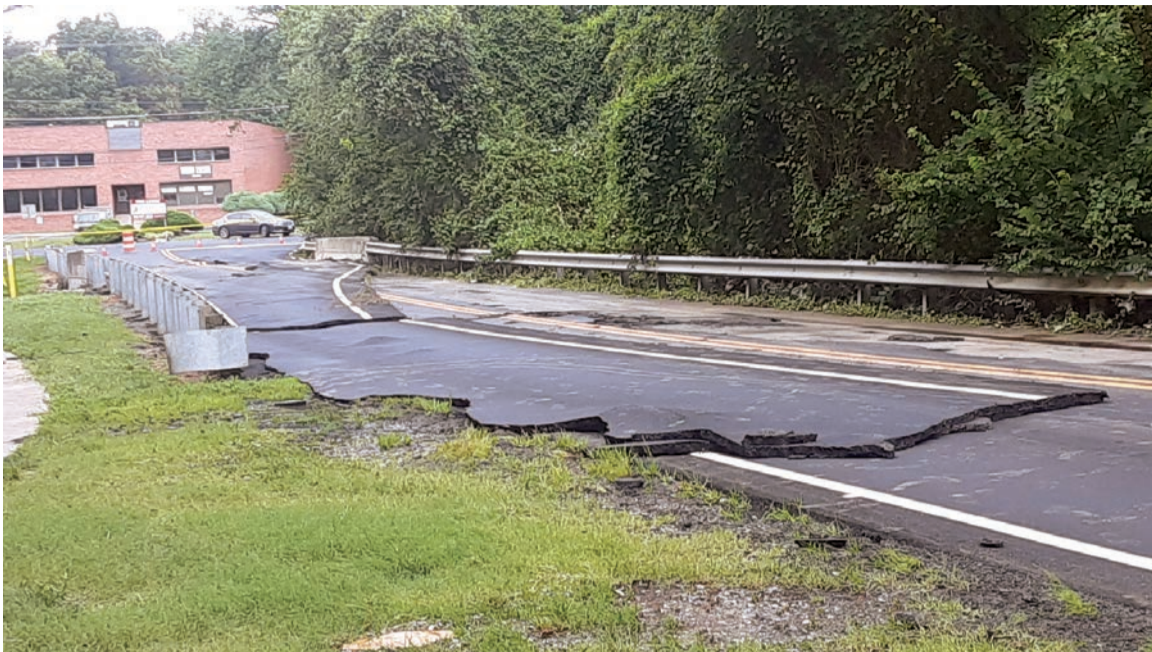
Water overflowed the banks of Long Branch and damaged newly-paved Newington Road.
