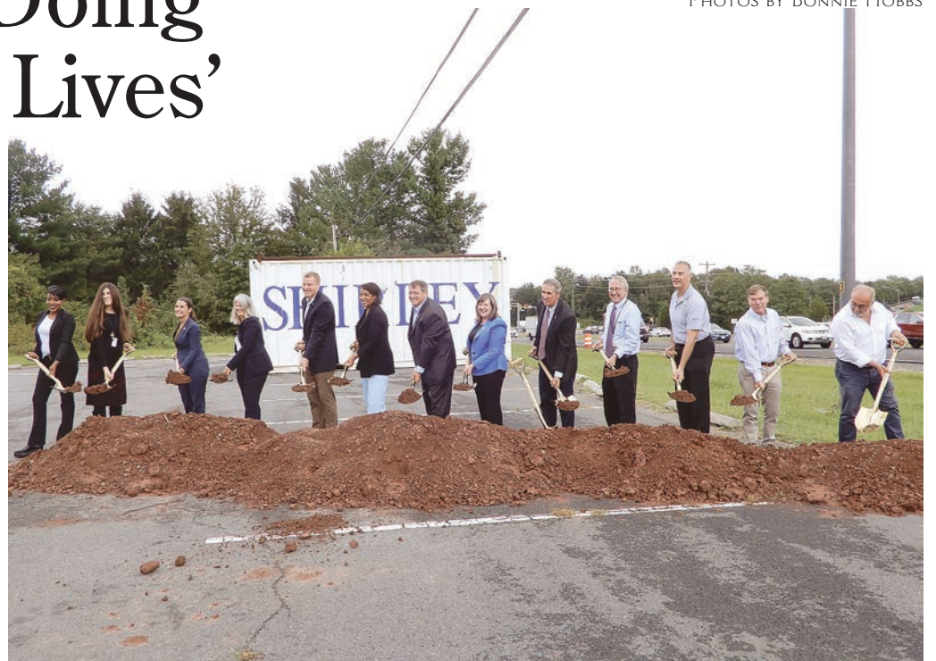
Officials break ground for the Route 28 widening. In the center are Jeff McKay, Phyllis Randall, Pat Herrity, Kathy Smith (blue jacket) and John Lynch. Del. Danica Roem and Sen. Jennifer Boysko are on the left.
