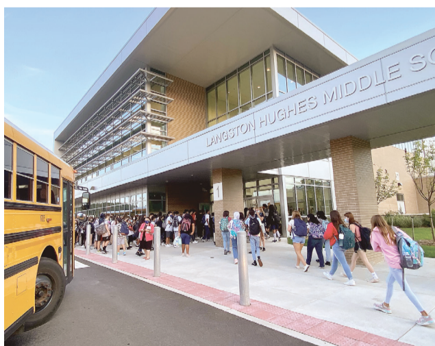
The $39 million renovation project at Langston Hughes Middle School in Reston welcomed students back to in-person learning in fall 2021 and added about 183,566 square feet to the school. Close-out work is anticipated to be completed by the end of 2021.
