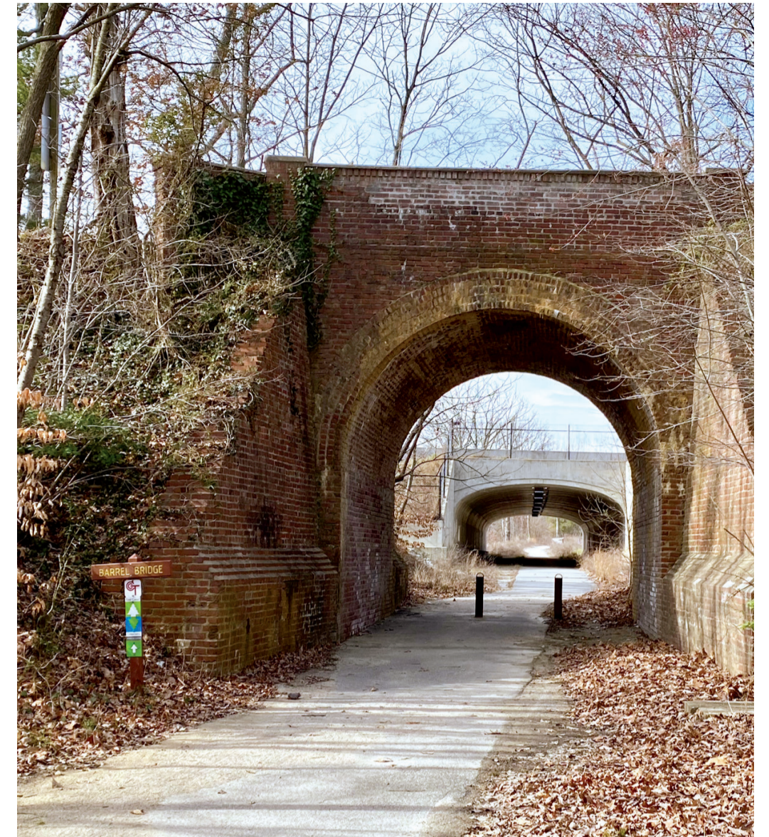
The historic Barrel Bridge, built by inmates, now serves cross county trail users where once a rail line moved materials across the Occoquan Workhouse/Lorton Prison grounds (March 2020).
