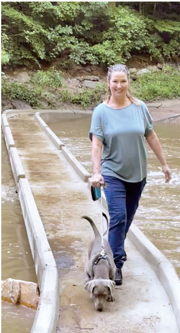
Stefie Pratt-Green and Levi use an improvement to the fair-weather crossing on the Pohick Stream portion of Gerry Connolly Cross County Trail. (June 2021)
