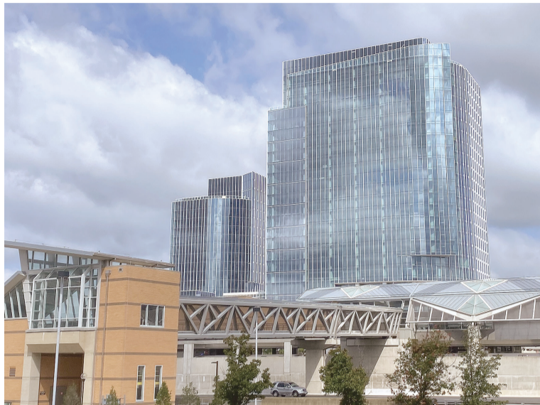
A view of the new pedestrian walkway over the Dulles Toll Road that accesses Metro's Reston Town Center Station and joins the 14-acre Reston Crossing Development located south of the toll road between Edmund Halley Drive and Reston Parkway.
