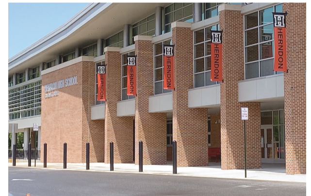
Herndon High School renovation at the cost of $83.9 million and designed by Hughs Group Architects added more than 138,558 square feet to the building constructed in 1980 and expanded capacity for 2,500 students. Work should be completed by summer 2022.
