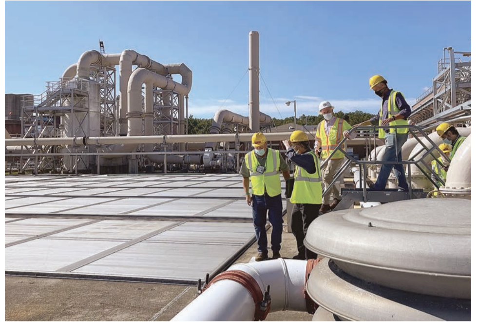
Virginia Master Naturalists observe the Grit Train mechanism that removes materials heavier than water which are hauled to the landfill.
