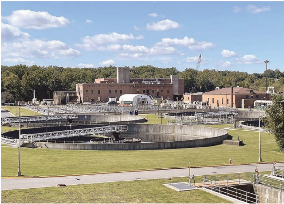
The Noman Cole Jr. Pollution Control Plant, celebrated 50 years of service in 2020.
