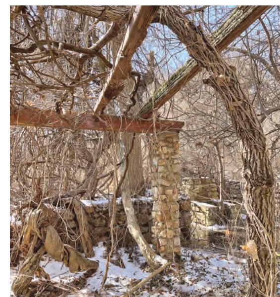
An 8-column quartz pergola and brick barbecue are just visible in one tier of the garden through extensive vine growth and fallen trees.
