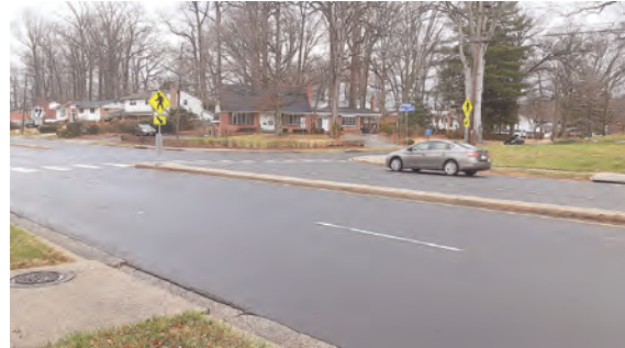
Looking across Burke Lake Road, this crosswalk will be part of the improvements to Braddock Road.
