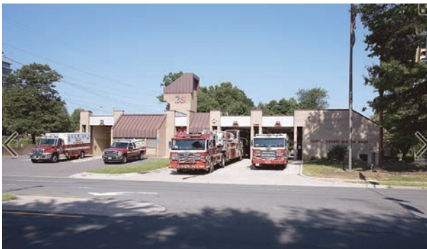
The original building of Fairfax County Fire and Rescue Station 25, Reston located at 1820 Wiehle Ave. in Reston was built in 1972.
