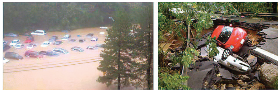
Figure 3. (Left) Tropical Storm Lee flooded Reston Park and Ride facility in Fairfax County (Source: weather.gov, courtesy of NBC Washington); (Right) Tropical Storm Lee damaged Lorton Road in Fairfax County (Source: Virginia Department of Transportation).
