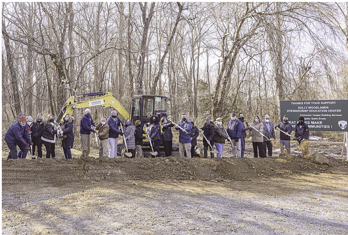
Local dignitaries and stakeholders break ground on the Sully Woodlands Stewardship Education Center. Supervisor Kathy Smith (D-Sully) is in the plaid coat.
