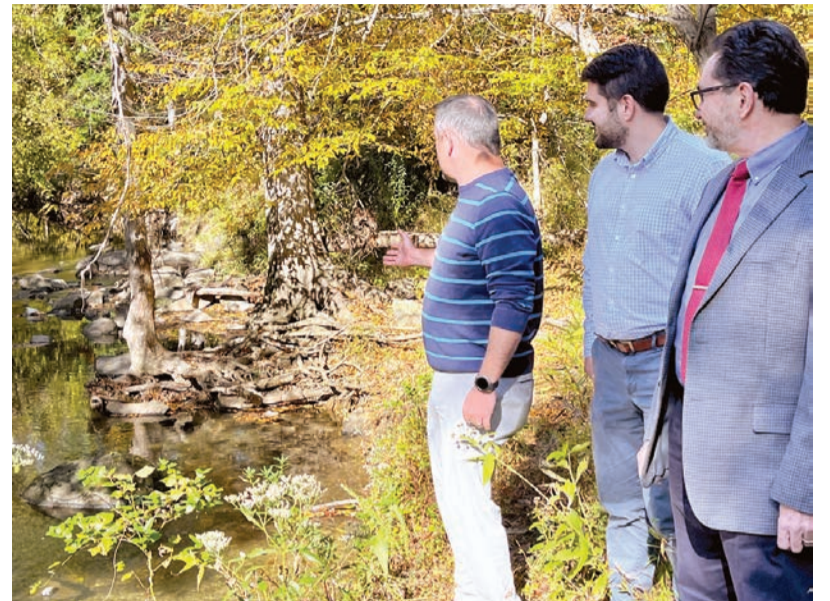
Richard Smith, a senior civil engineer; Lawrence Latour, PE, water resource engineer; and Scott Robinson, director of public works; all with the Town of Herndon, look at the Sugarland Run’s bed and bank erosion.
