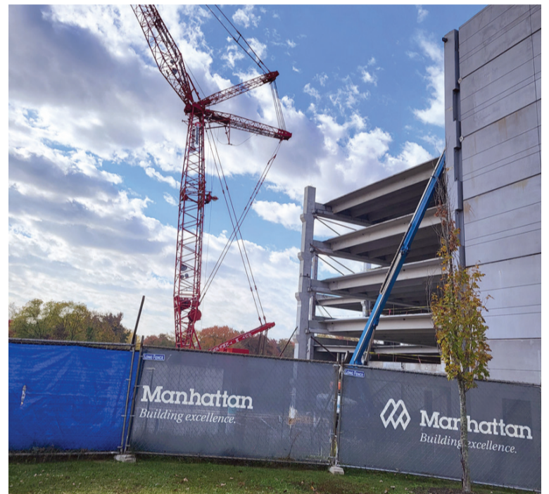
A crane towers over the new paved areas behind the structure.
