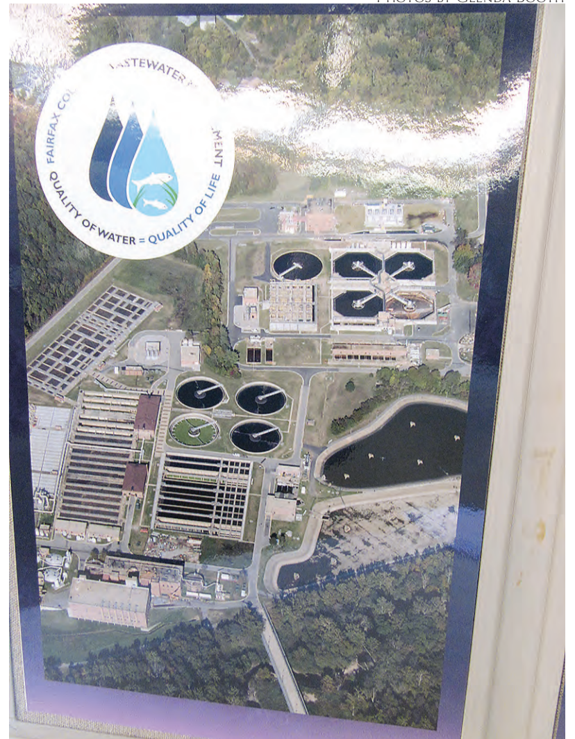
Overhead view of the Noman Cole plant, a poster on display there.
