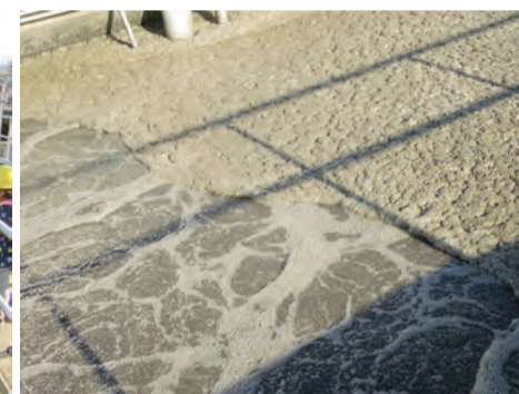
This wastewater is undergoing secondary or biological treatment using bacteria.
