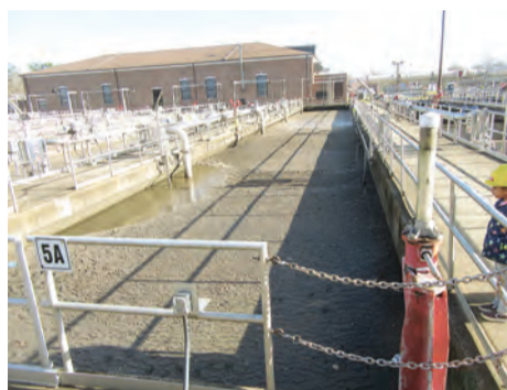
This wastewater is undergoing secondary or biological treatment using bacteria.
