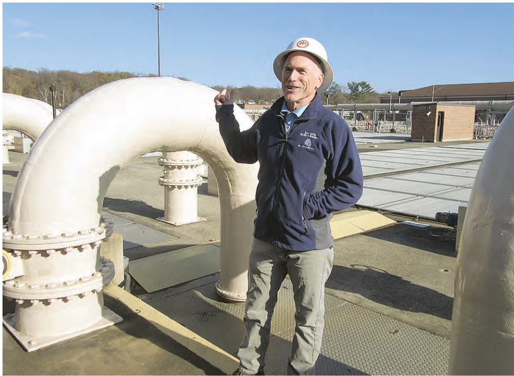
Mike McGrath, Director of Wastewater Treatment, explains primary treatment at a settling tank.
