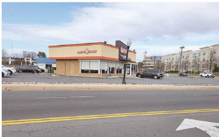
This Dunkin Donuts around the corner is relocating to the newly refurbished site a block away.
