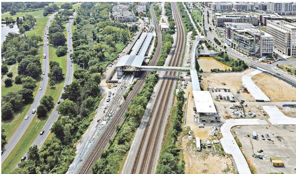
Aerial view of Potomac Yard construction, with the long delayed station now scheduled to open May 19.
