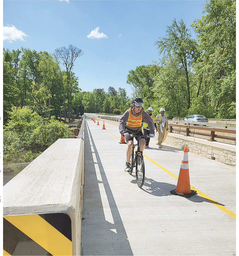
This new bridge over Dogue Creek is a connector to the Mount Vernon Trail on the southern end.
