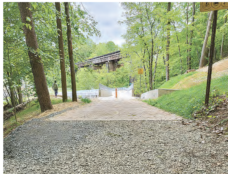
Looking north down on the new bridge.
