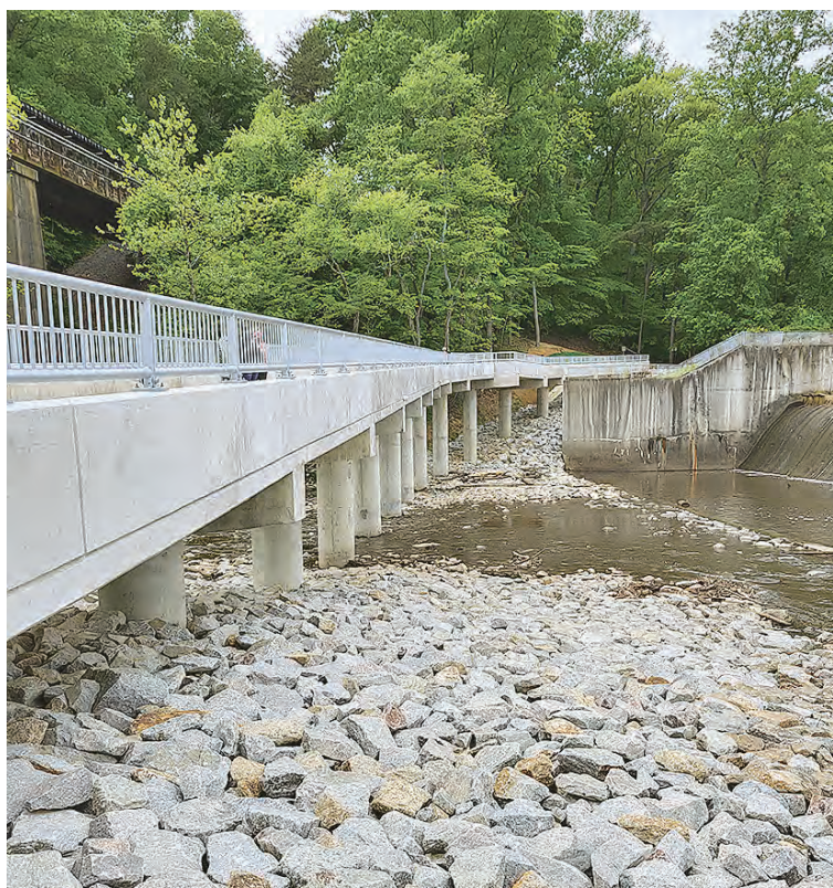
The new bridge clears the spillway.
