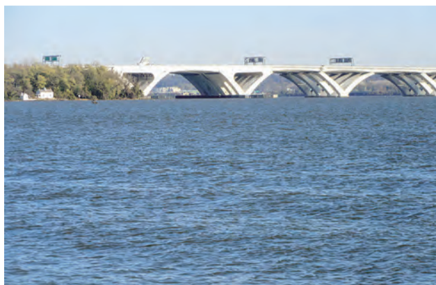
The Woodrow Wilson Bridge spans the Potomac River, connecting Virginia and Maryland.
